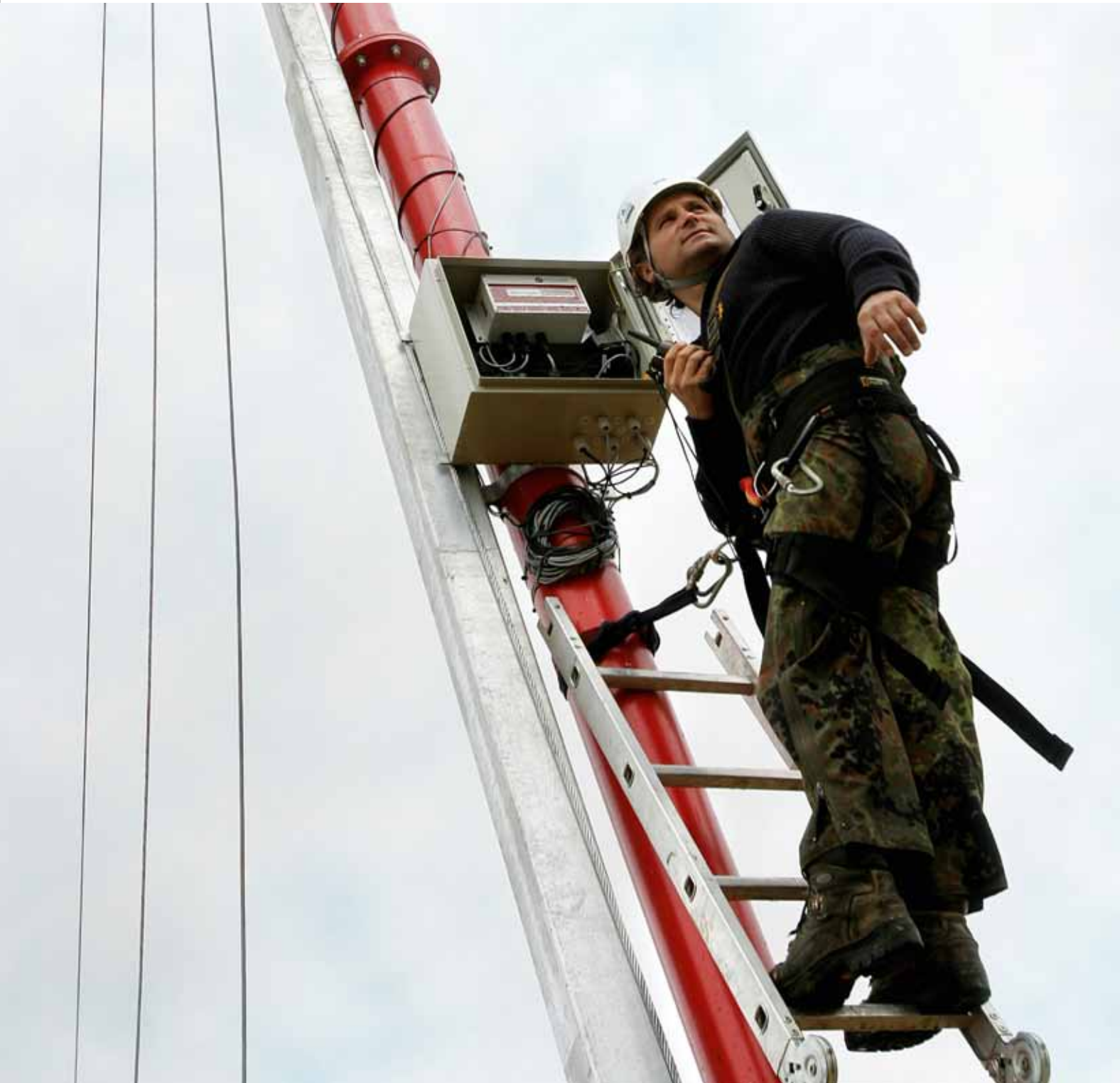
© Ammonit / Windhunter (Ammonit partner Poland): logger, steel cabinet and logger accessories
